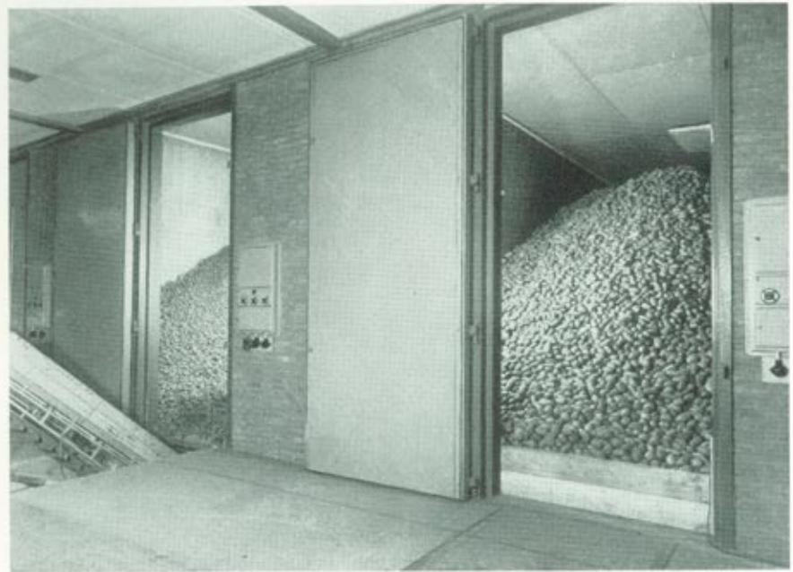
The insulated chambers permit the storage of several thousand tons and facilitate the receipt and dispatch at all times, even during frosty weather. Each of the 30 chambers contain approximately 80 tons of potatoes and are equipped with refrigeration and ventilation. A special feature of the cooling equipment is the thermostatic control operated from one central point, installed by Unitem.
